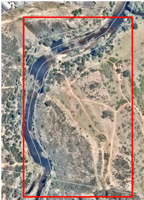
Aerial photo showing area of interest located in the southwestern corner of the proposed Jumping Creek development
